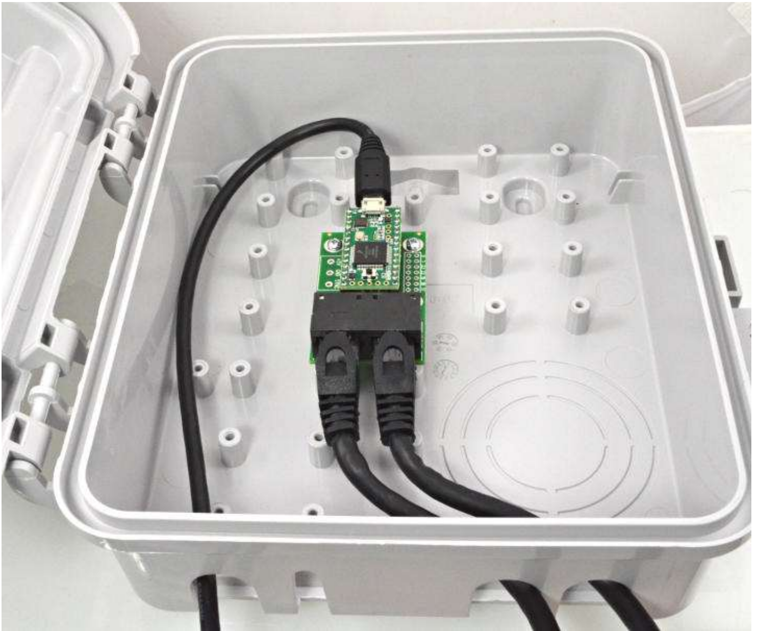
The eight LED outputs are sent on two CAT6 Ethernet cables.
